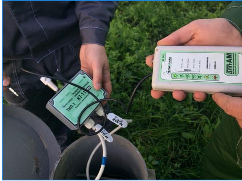
Pipeline monitoring today
